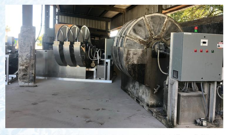
The Rotary Disc Vacuum System by ESD Waste 2 Water Inc. is designed to reduce moisture content in sludge by 85% or more. The RDV produces a cake material that can be easily transported for disposal.
